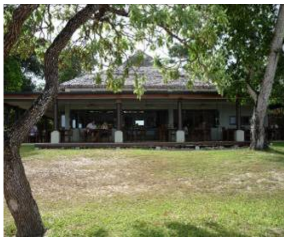
Erap-Lodge: View of the main hall of the lodge
