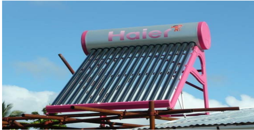
A Name Brand Flooded Evacuated Tube Solar Water Heater (Tonga)
